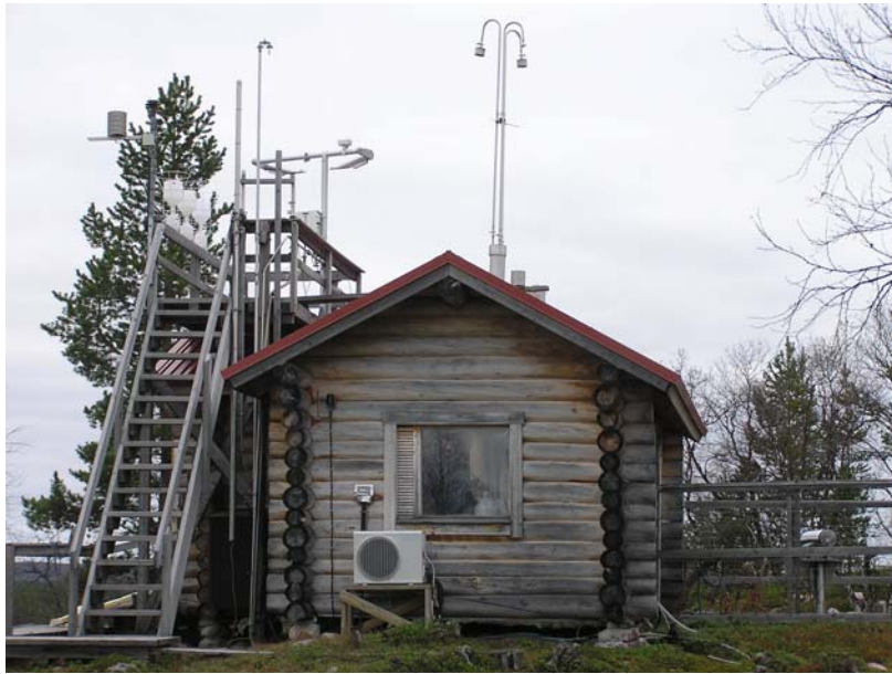
Fig. 2. Sevettijärvi air quality monitoring station.
